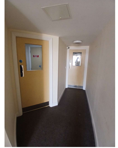
Internal Doors (Compartment Doors)
